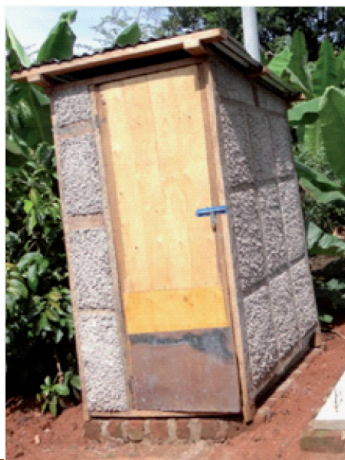
Figure 8: Superstructure made of ferrocement
