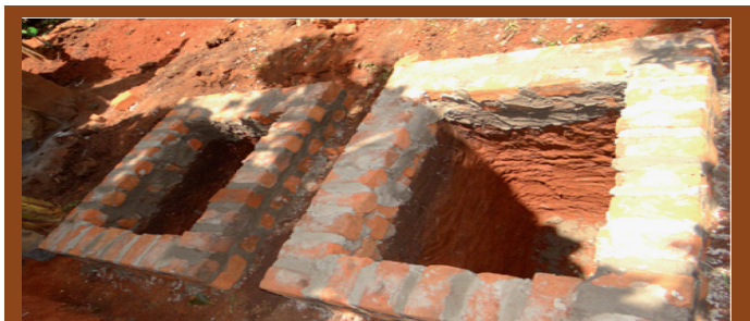
Figure 3: Construction of ring beam using bricks
