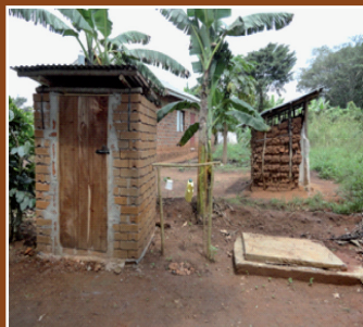
Figure 9: Demolishable superstructure constructed using ISSB (left) and two pits in one superstructure (right) constructed using ordinary burnt bricks
