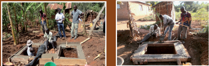
Figure 2: Construction of ring beams using steel bars
